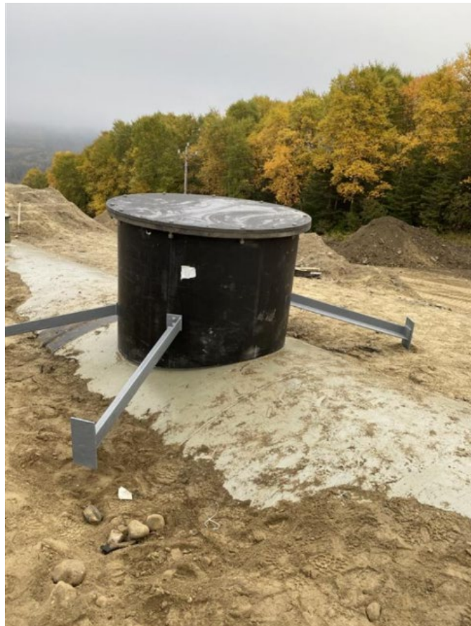
Figure 1: New Access Cover Installation
