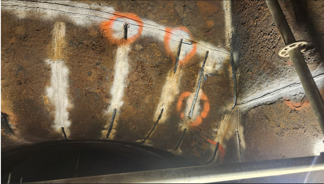
Figure 2: Weld Repairs at Surge Tank Transition
