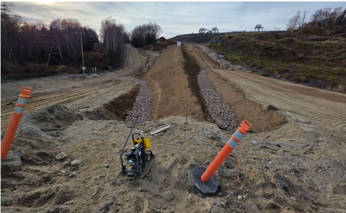
Figure 7: General Penstock Backfill and Final Grading
