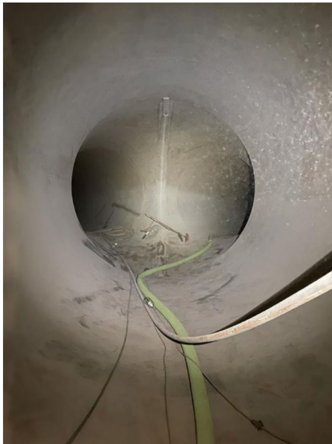
Figure 3: Sandblasting and Cleanup at the Bifurcation
